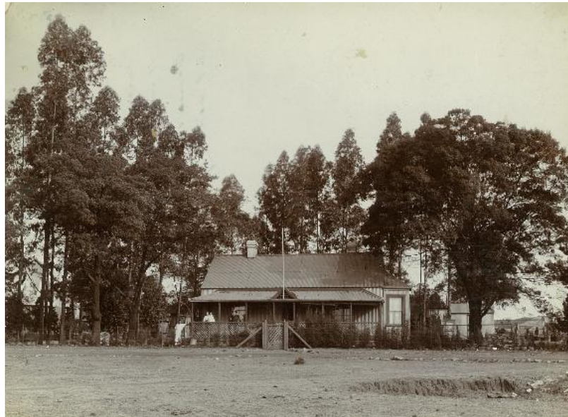
Resident Engineer's House – Crown Reef - 1904
